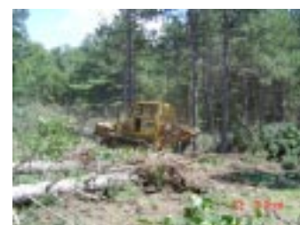
Reducing woody cover using a bulldozer
